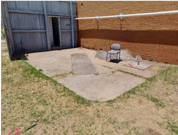
View to the south-east of a filled inspection pit
