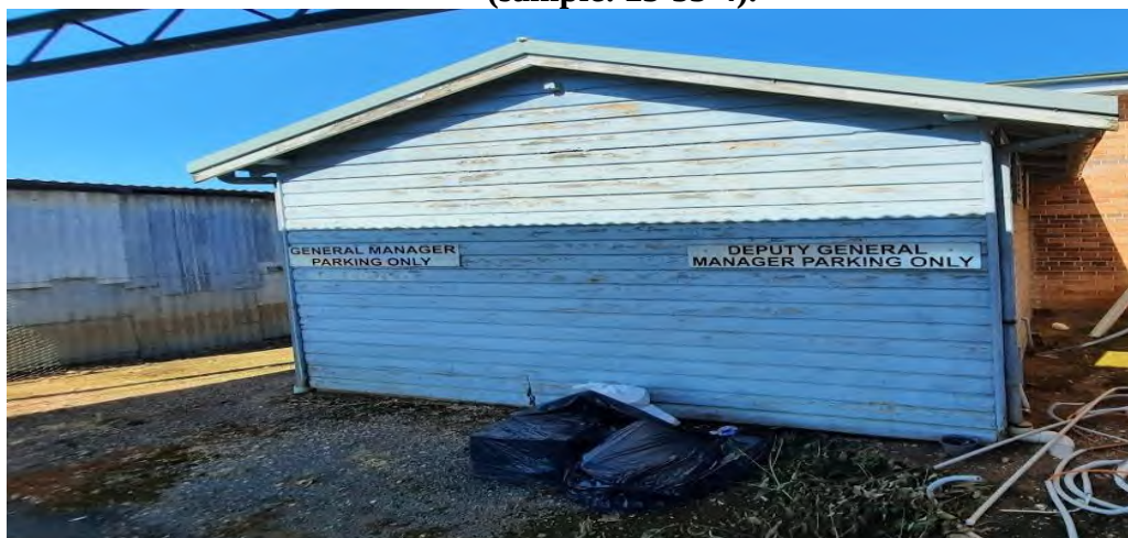
Figure 13: Confirmed lead base paint on the walls and topsoil around the toilet building (sample: 23-33-4).
