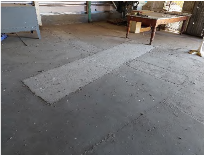
View of sealed inspection pit at the workshop area
