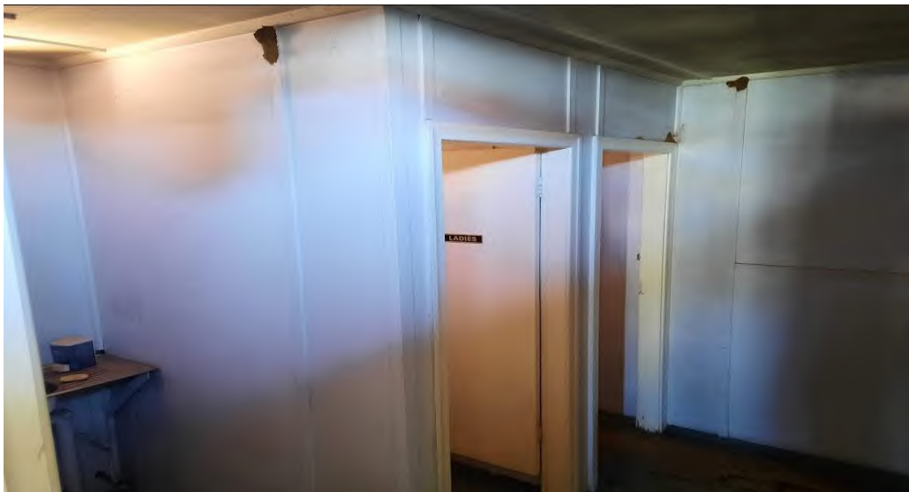
Figure 13: Confirmed lead base paint on the walls and topsoil around the toilet building (sample: 23-33-4).
