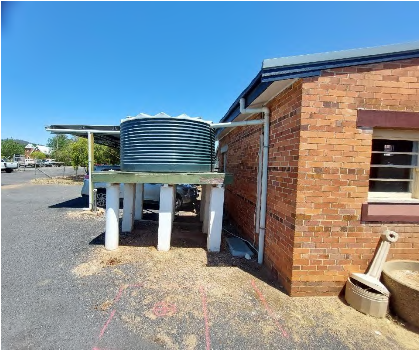
Photograph 4 View to the south of the stormwater tank
