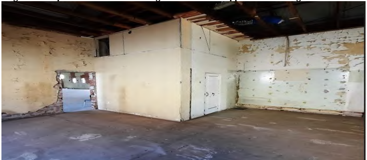
Figure 9: Suspected asbestos containing material on the upper wall sheeting of the storeroom.
