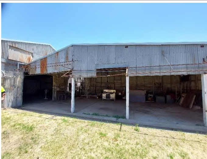
View to the north of the workshop area
