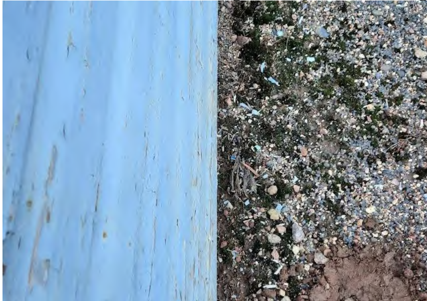
Figure 10: Paint flakes scattered on the ground adjacent to a flaking painted wall.
